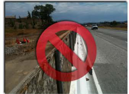
Protect workers and work sites
